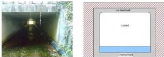
Figure 4 - Simple Culvert - Box
